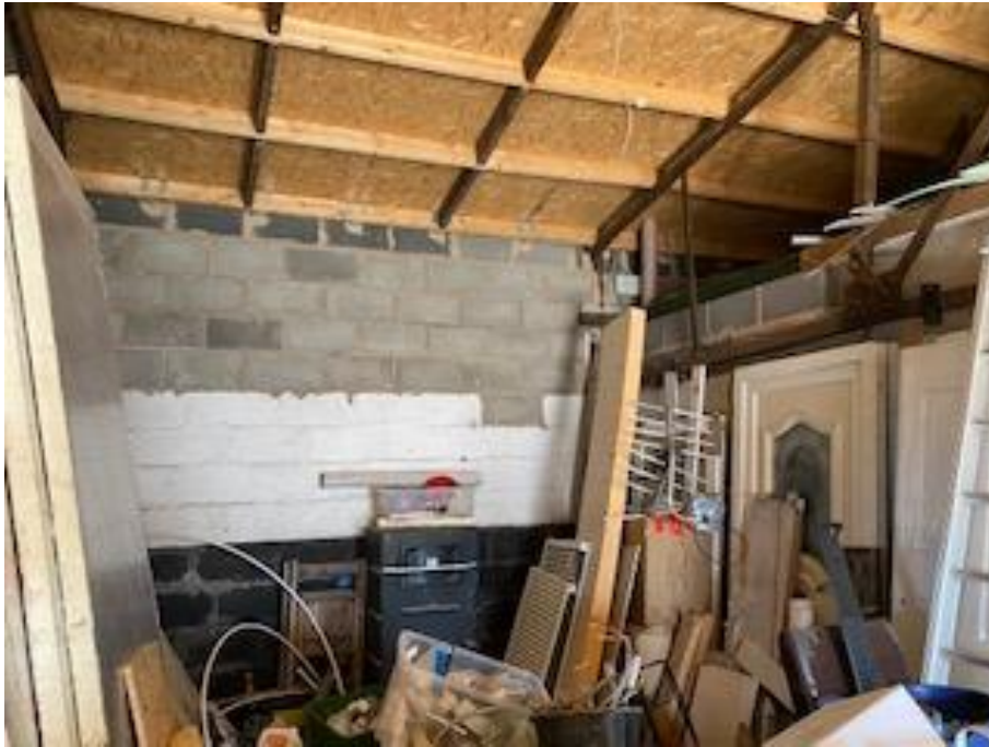
Photo 3 this is the would be 'snug area' after renovation
